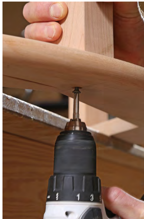
Drive the screws. With the table upside down, Coleman drives the screws \frac{1}{4} in. to \frac{1}{2} in. into each leg to make sure they don't move while he drills for and drives the dowels.
