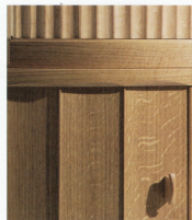
Defining details. Subtle scallops in the lower edge of the waist molding reflect the graduated curves of the doors below.
